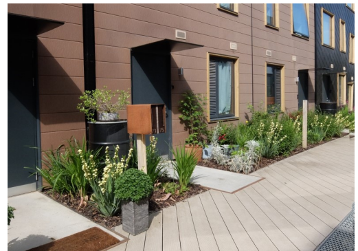
The CITU Climate Innovation District development in Leeds City Centre. Low carbon, factory made homes designed for their location
