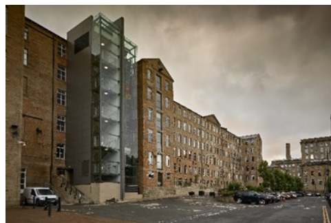
A Mill, right, and B Mill, showing the new, glazed lift and stair tower alongside the redundant stair and loading tower, now turned into meeting rooms.
