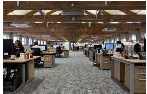
Top-floor, open-plan office space, showing the cleaned and exposed roof trusses.
